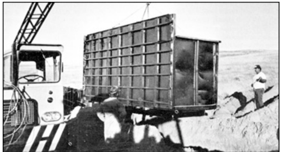
Bill Ewert watches section being lowered into place.
